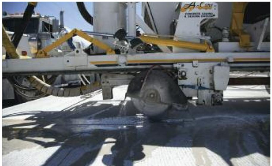
**How'd we do it?** We did it with great people and innovative equipment. Once again, A-Core deployed the state-of-the-art Spider Saw. This saw consists of a mechanical arm that spins multiple blades a onetime which, allows for one single operator to cut a transverse joint in seconds, resulting in higher production. This machine substantially increases cut time, making possible for A-Core
